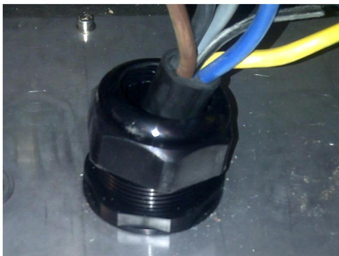
1. Slide the cable gland(s) over the cable(s).
