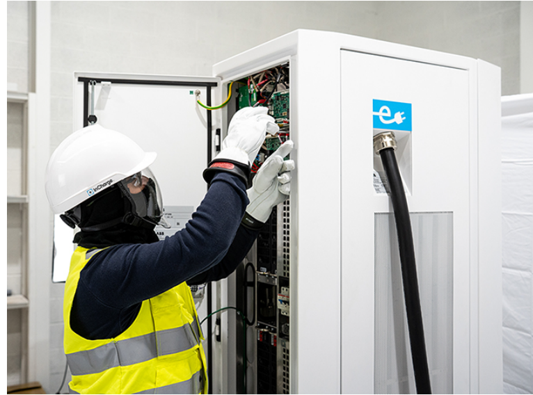
InCharge technician servicing an ABB Terra DC Fast charger.
