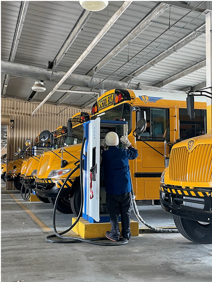
InCharge technician servicing an ICE-60 DC Fast charger.
